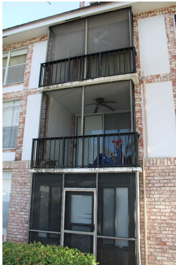
Photograph 2 – Typical view of the balconies and railing system.
