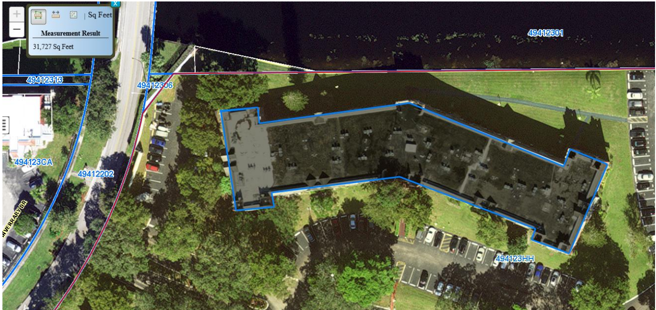
Figure 2: This image, sourced from the Broward County Property Appraiser, displays the footprint of the building located at 3760 Inverrary Drive, Lauderdale, FL 33319.
