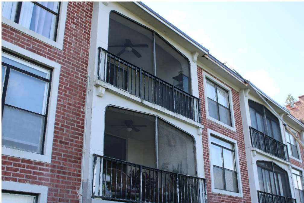
Photograph 4 - Typical view of windows system, balconies and decorative wooden features.
