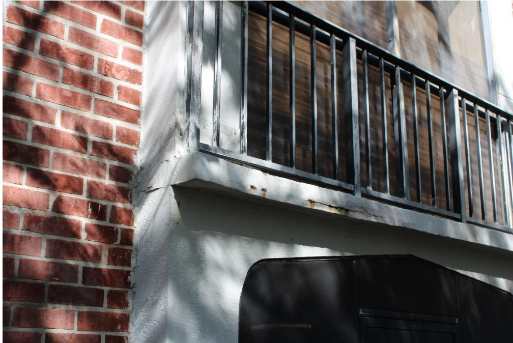
Photograph 3 - View of the building envelop, featuring a stucco finish combined with decorative stone cladding.
