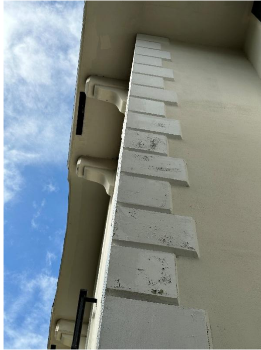
Photograph 3 - View of the building envelop, featuring a stucco finish combined with decorative stone cladding.
