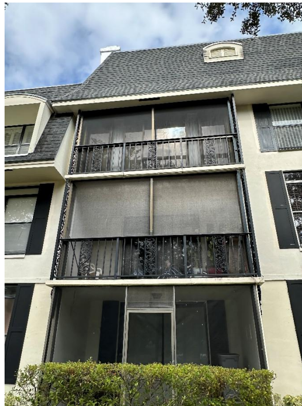
Photograph 2 - Typical view of the balconies and railing system.
