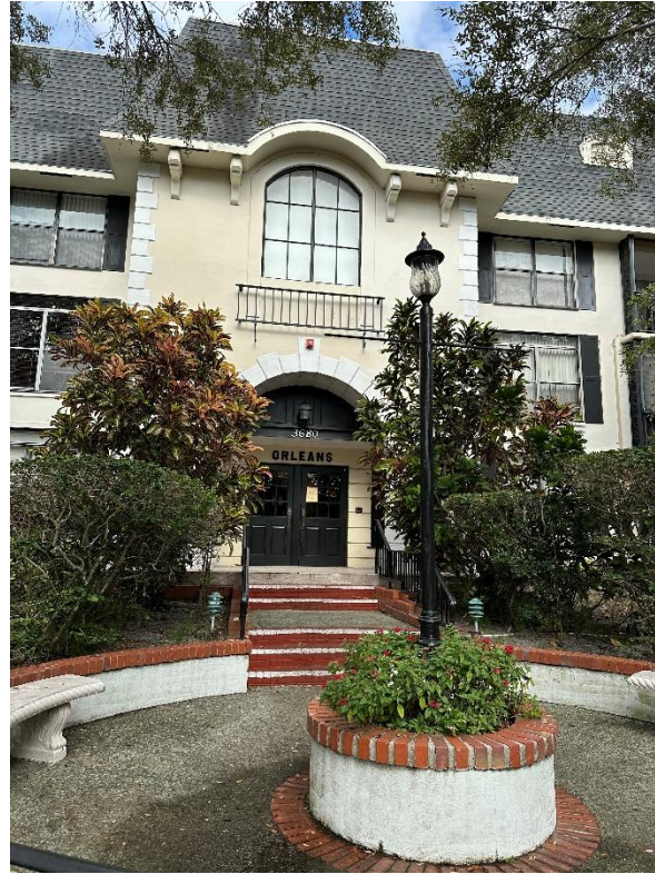
Photograph 1 - View of the main entrance.
