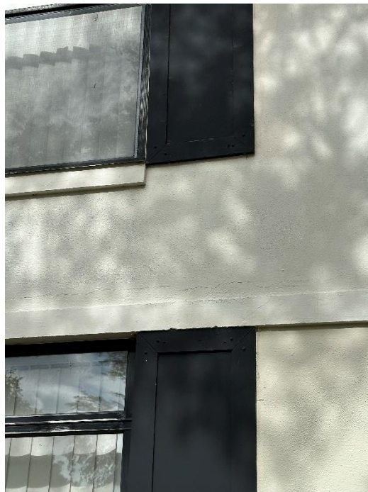
Photograph 4 - Typical view of windows system and decorative wooden features.
