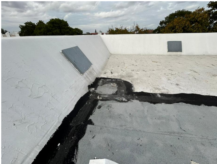
Photograph 8 – View of the Mansard roof sections.
