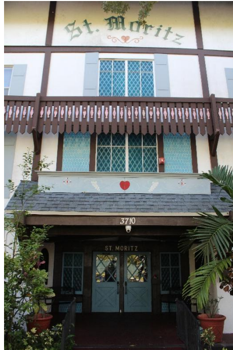
Photograph 1 - View of the main entrance.
