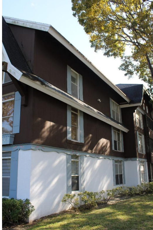
Photograph 3 - View of the building envelop, featuring a stucco finish combined with decorative wooden cladding.
