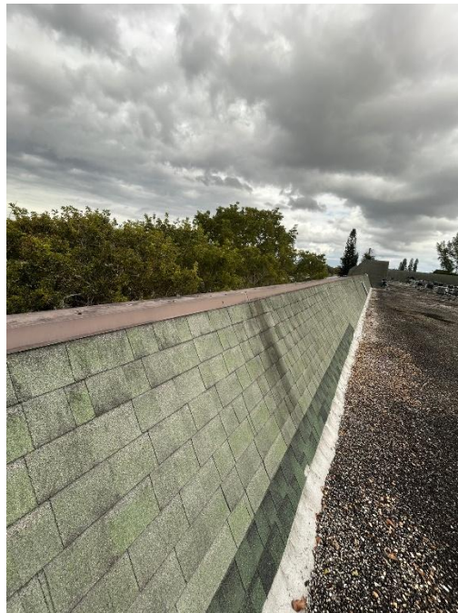
Photograph 6 – View of Mansard Roof.
