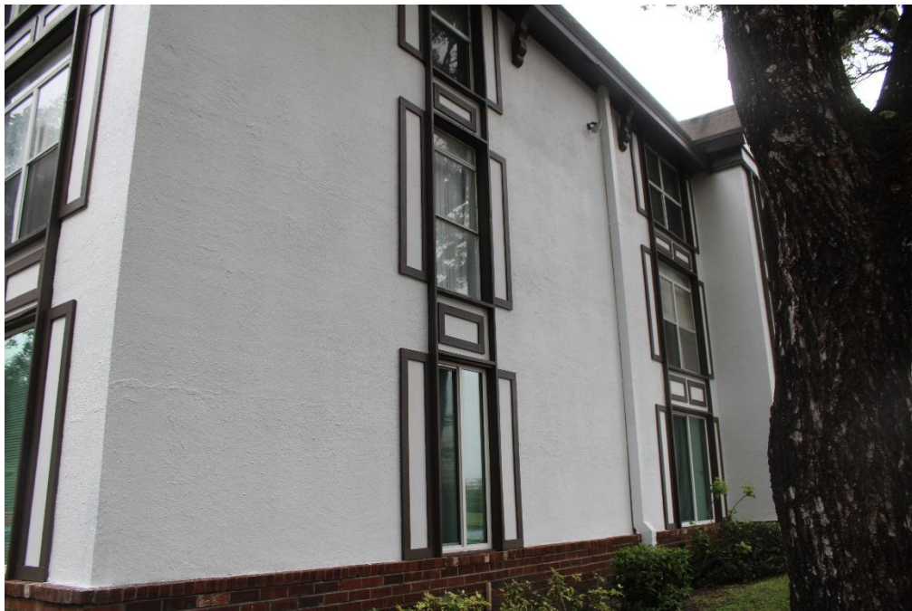
Photograph 4 - Typical view of windows system and decorative wooden features.
