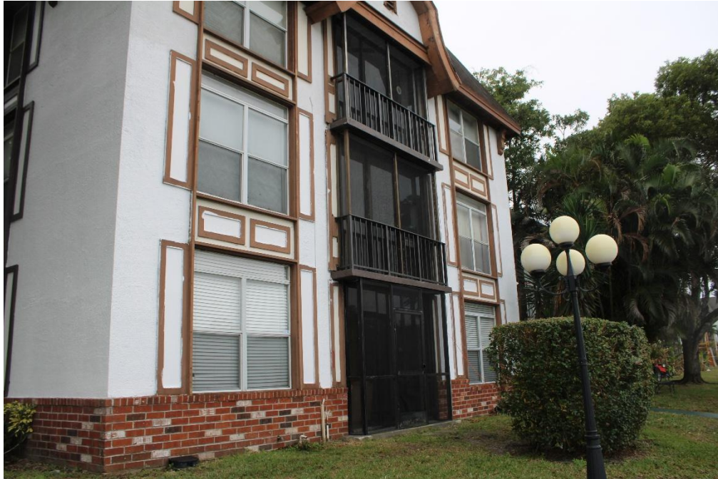
Photograph 3 - View of the building envelop, featuring a stucco finish combined with decorative stone cladding.
