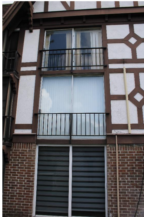
Photograph 4 - Typical view of windows system, balconies and decorative wooden features.
