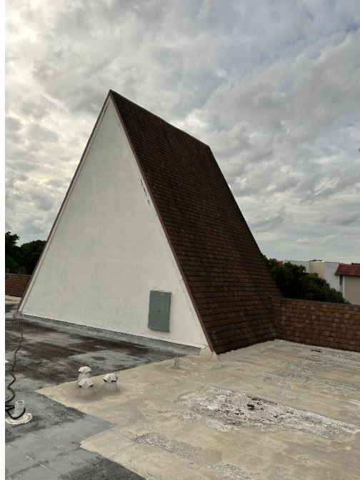
Photograph 7 - View of Mansard Roof.
