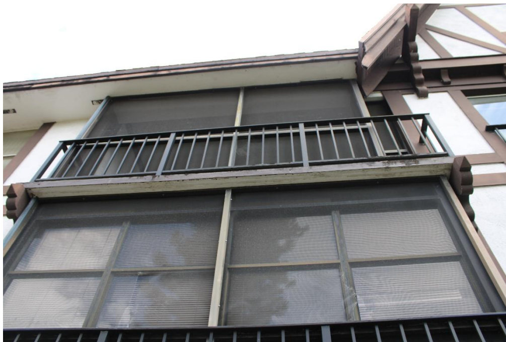
Photograph 2 - Typical view of the balconies and railing system.
