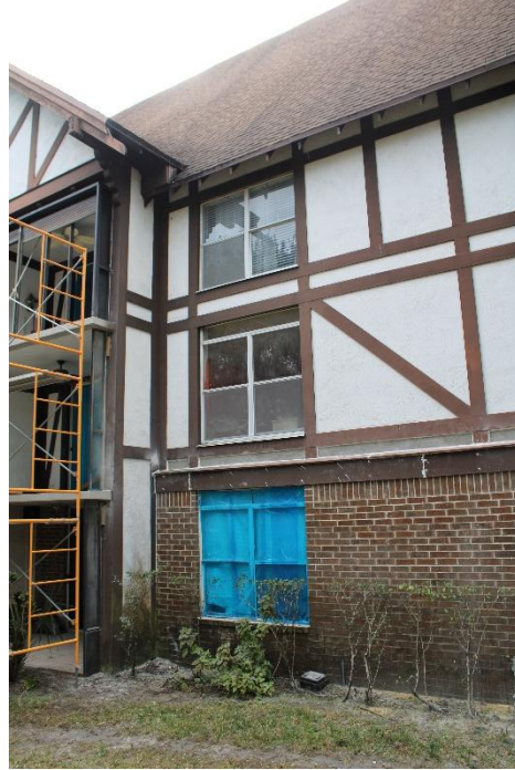
Photograph 3 - View of the building envelop, featuring a stucco finish combined with decorative stone cladding.
