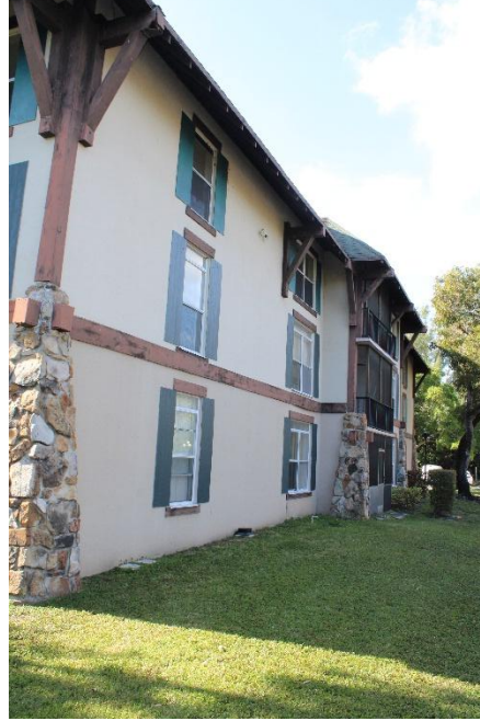
Photograph 5 – Typical view of window glassing.
