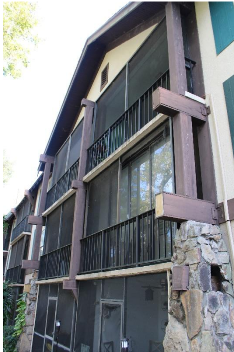
Photograph 2 – Typical view of balconies and architectural wooden accents.
