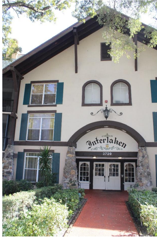
Photograph 1 – View of the entrance of the building.
